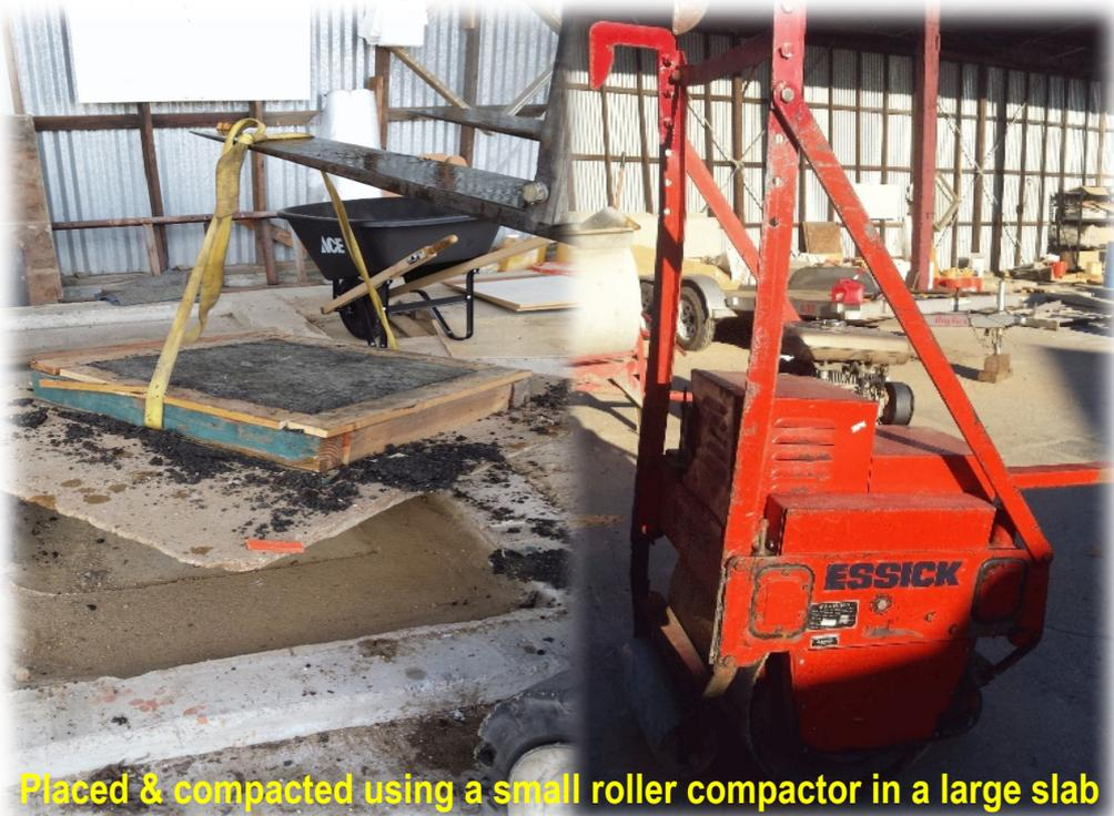
Placed & compacted using a small roller compactor in a large slab
